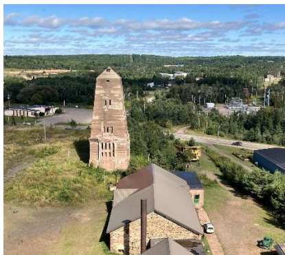
1 View from C shaft, hoist motors on same level as nest box, A and B shafts
